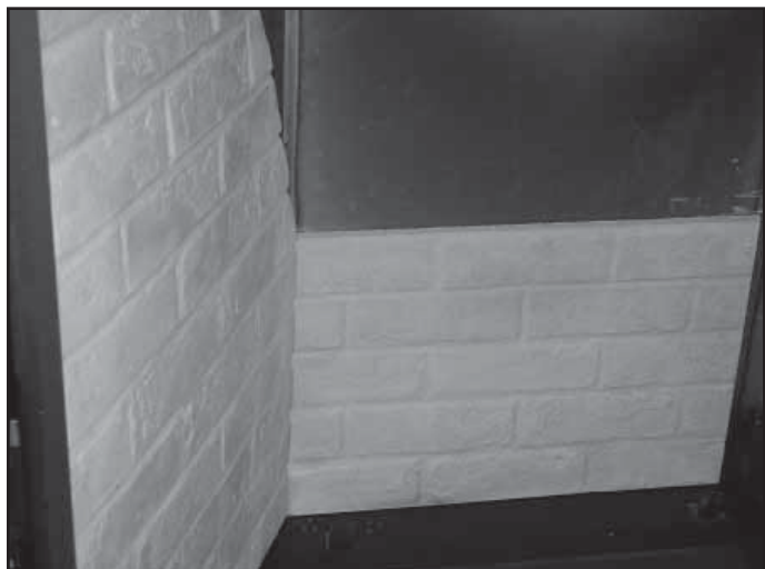
Figure 15.2 Install Lower Back Refractory
